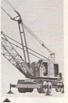
SPECIAL "HI-LITE" BOOM GANTRY is required for "HI-LITE" booms over 130 feet long to increase the angle of support between boom-hoist cables and boom, thereby reduc-
